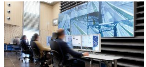
CCTV control room using rear projection cubes
