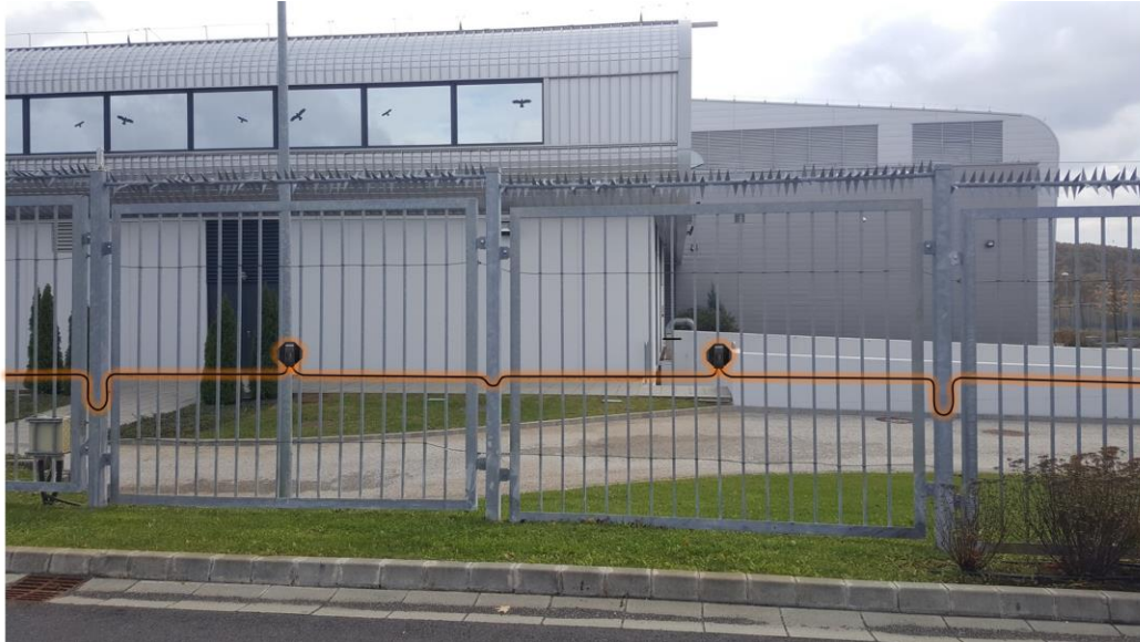
Pic. 2 – Detectors fitting example
